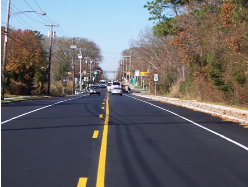
PHOTO 1: PAVEMENT AT 5.0 CRACK RATING (IMAGE TAKEN FROM IDAHO RATING MANUAL):
