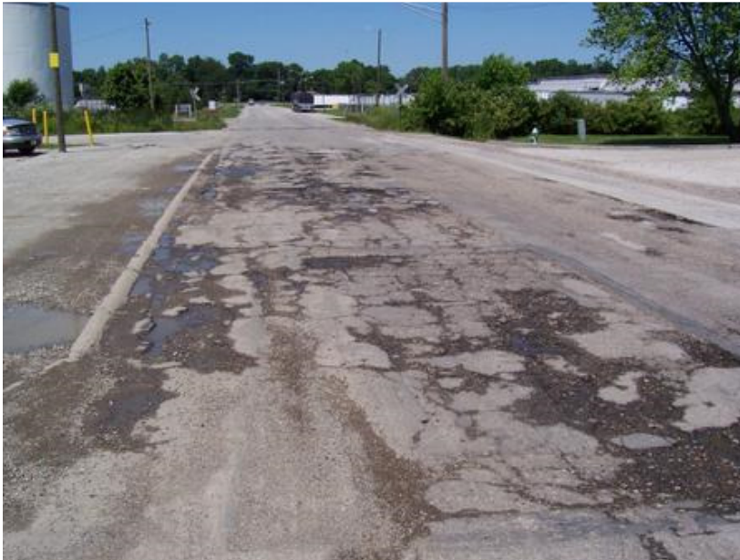
PHOTO 2: PAVEMENT AT 0.0 CRACK RATING (IMAGE TAKEN FROM IDAHO RATING MANUAL):
